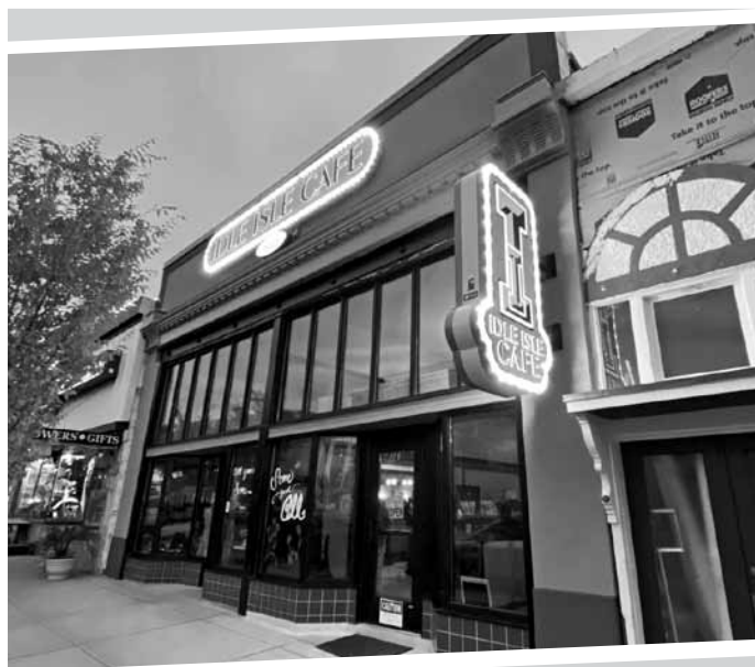
Idle Isle Cafe, Brigham City, Utah. 2021. Main Street revitalization allows rural towns to preserve historic storefronts and community character for locals and tourists alike. Image courtesy Brigham City Corporation.
