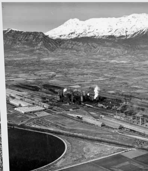
Geneva Steel Plant on the shore of Utah Lake, c 1945. Image courtesy Utah Historical Society.
