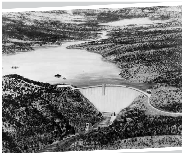
Flaming Gorge Dam and Power Plant, Artist's Conception, c 1955. The federal Bureau of Reclamation directed considerable investment into dams and diversions that store water, generate power, and provide for recreation. Image courtesy Utah Historical Society.
